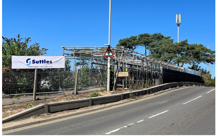
Figure 3: The footbridge from the road side
